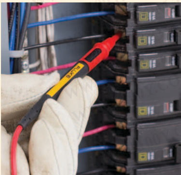
Reduce tip exposure for CAT III testing
