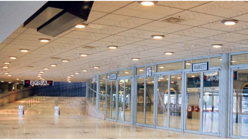
Electronic control gear from OSRAM provide greater comfort, economy and reliability in a large number of modern lighting solutions.
