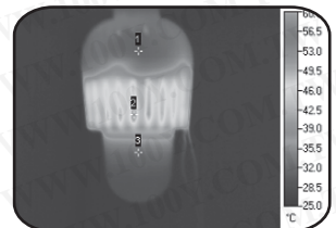
IR thermograph inspect
