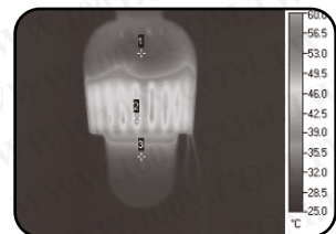
IR thermograph inspect
