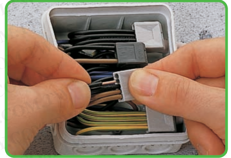
Termination: Insert stripped solid conductor fully.
