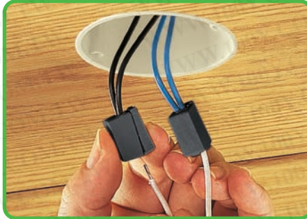
To connect: Press button fully and insert stripped conductor into square entry until it hits backstop and release.
